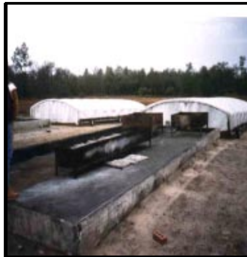
Closeup view of burning pans on concrete slab. Note the white covers in the background which can be rolled over the pans to prevent precipitation from entering them.
